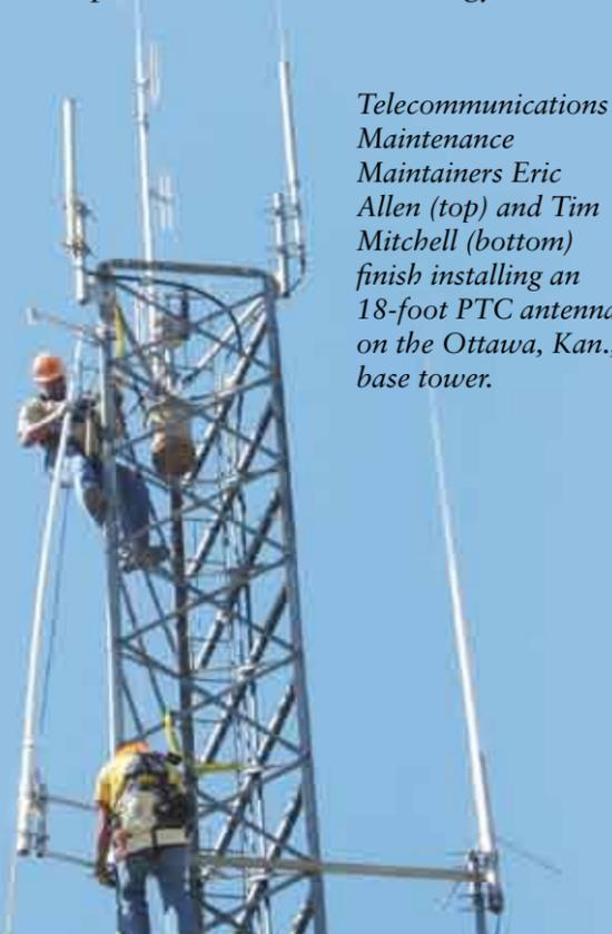
*Telecommunications Maintenance Maintainers Eric Allen (top) and Tim Mitchell (bottom) finish installing an 18-foot PTC antenna on the Ottawa, Kan., base tower.*
